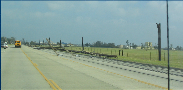
Long stretch of downed power poles along highway 14 in Lake Charles, Louisiana from Hurricane Rita. September 2005.
